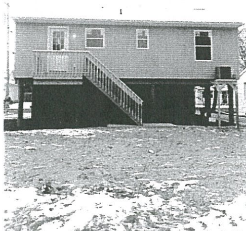
85 Illinois Avenue, Rear, 12/13/13
